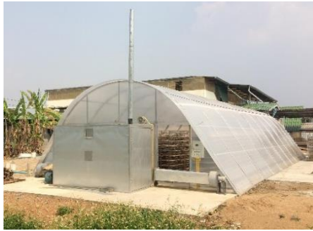
Figure 3 Solar dome with heat exchanger using biomass energy
